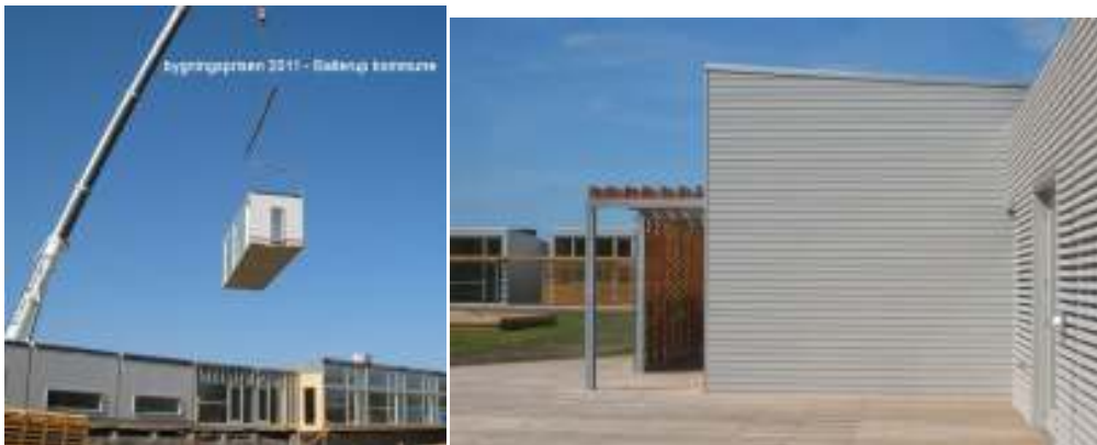
Montage of the modules.
